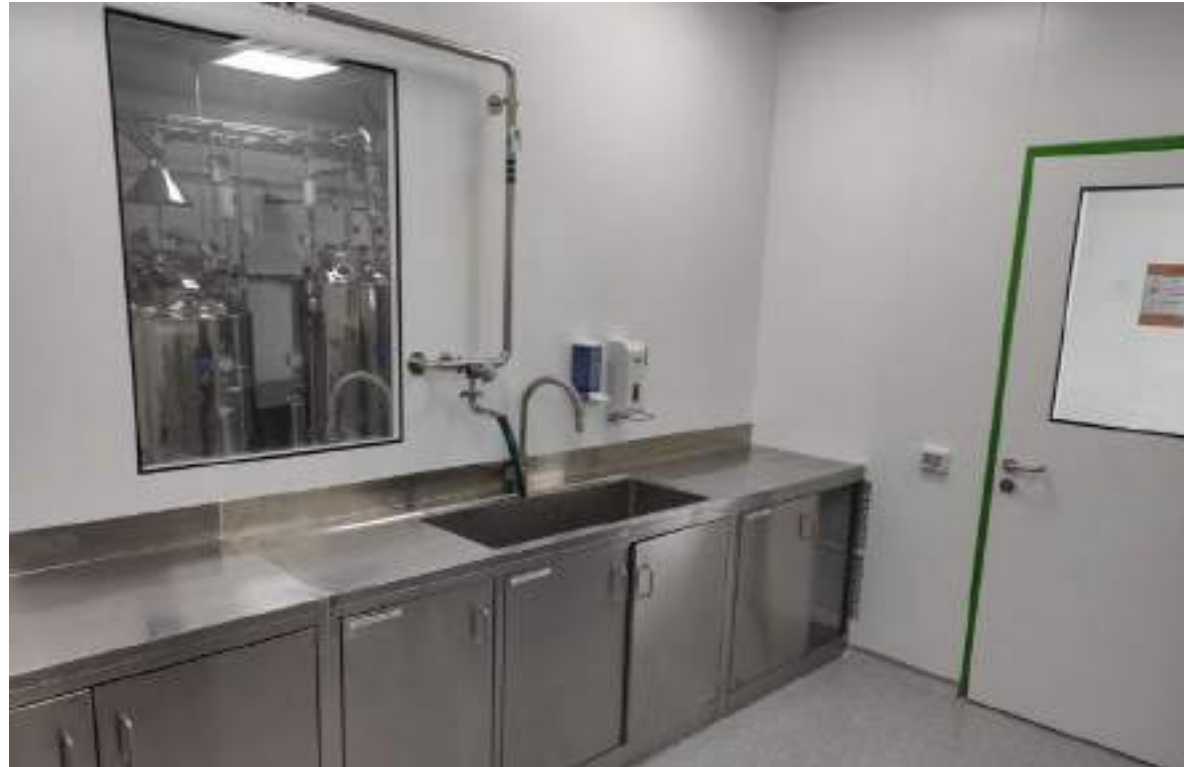
Sink area for components of VLZ bottling machines
